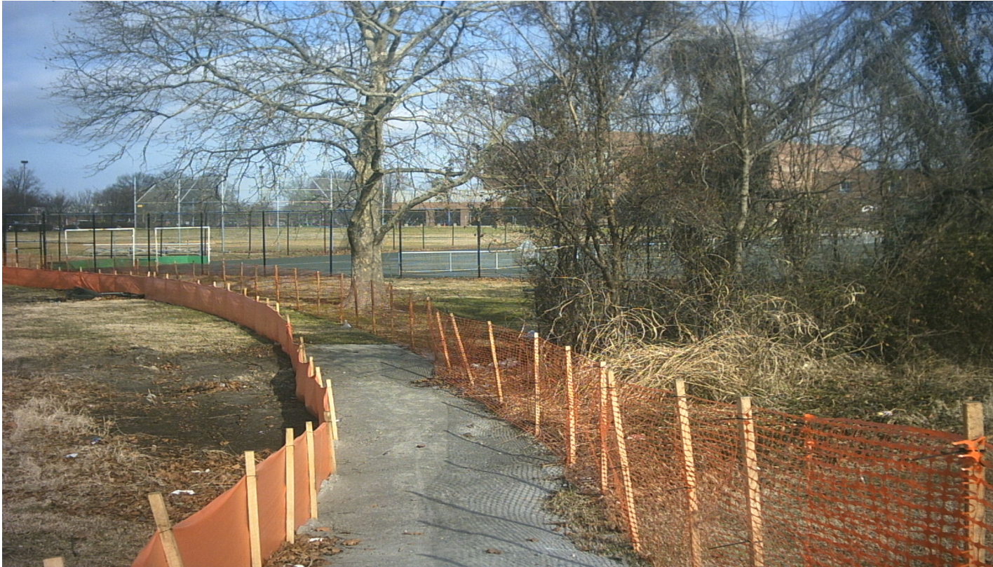
Temporary Walkway located at Holt Street
