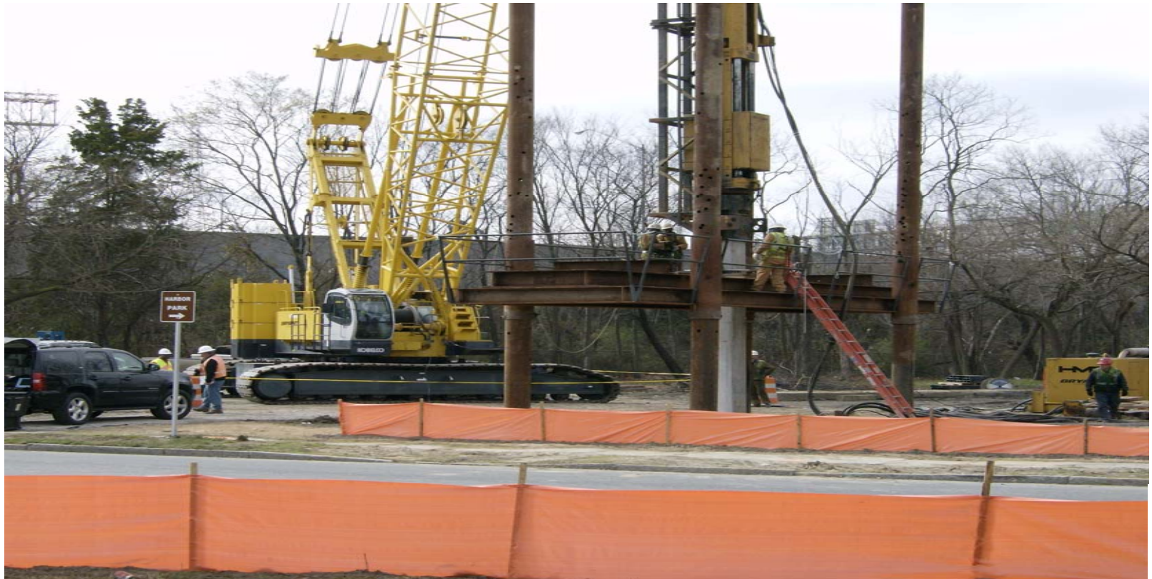
Test Pile Driving
